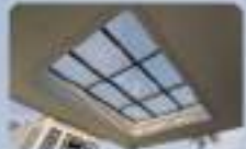
Canopy with Skylight
